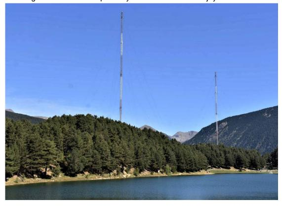
left: the 2 masts were linked to the Encamp transmitter by two 1km feeder lines. Last frequency being used before its closure in 1981 was 702 kHz.
