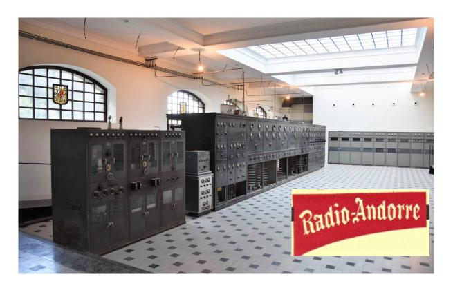
Above: Radio Andorra transmitter hall at Encamp with (left to right) SFR SW and MW transmitters dating to 1939, and on the far wall, the Brown Boveri MW transmitter from 1964.
