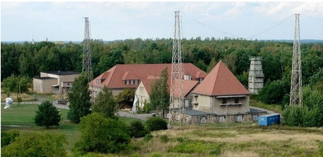
Above: Museum showing three remaining aerial towers (two on right still supporting a MW T-aerial). At the foot of the right hand tower is a trailer used to house a mobile 20 kW mediumwave reserve transmitter.
