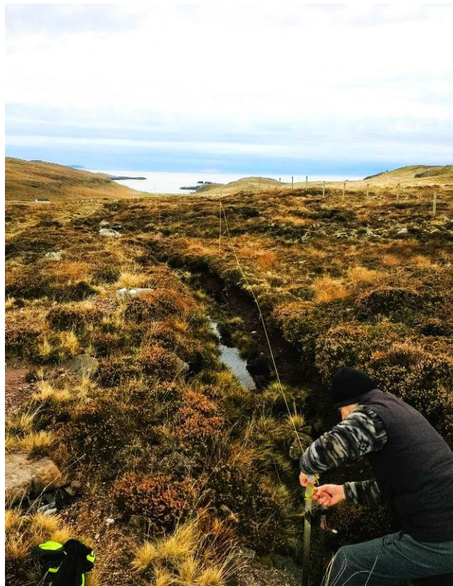
left: Dave fixes earth rod at end of 40° Beverage
