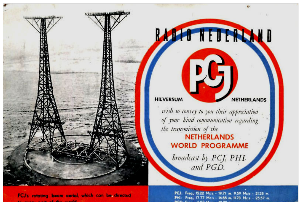
A Radio Nederland PCJ QSL from the late 1940s showing the remarkable wooden rotating beam aerials at Huizen. (They were constructed in 1937 and demolished in 1940)
